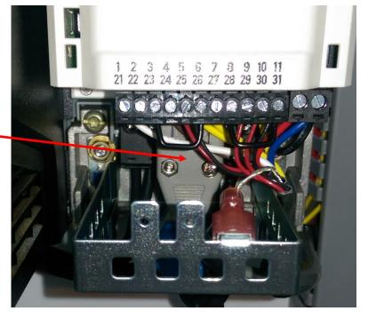
Slide the left side of the grounding bracket UNDER the ground lug and push up to the stud.
