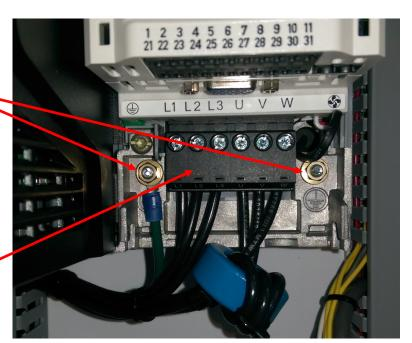
Re-install connector and secure with both side screws.
