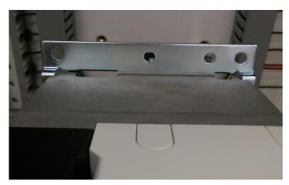
Reattach the ground lug and both nuts. Do not tighten yet.
