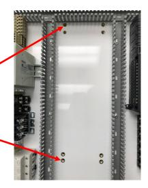
If the back panel has four nut inserts (two at the top and two at the bottom), a conversion bracket for the bottom two inserts will be required.
