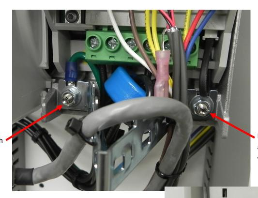
Remove nut using a 5/16" socket wrench
